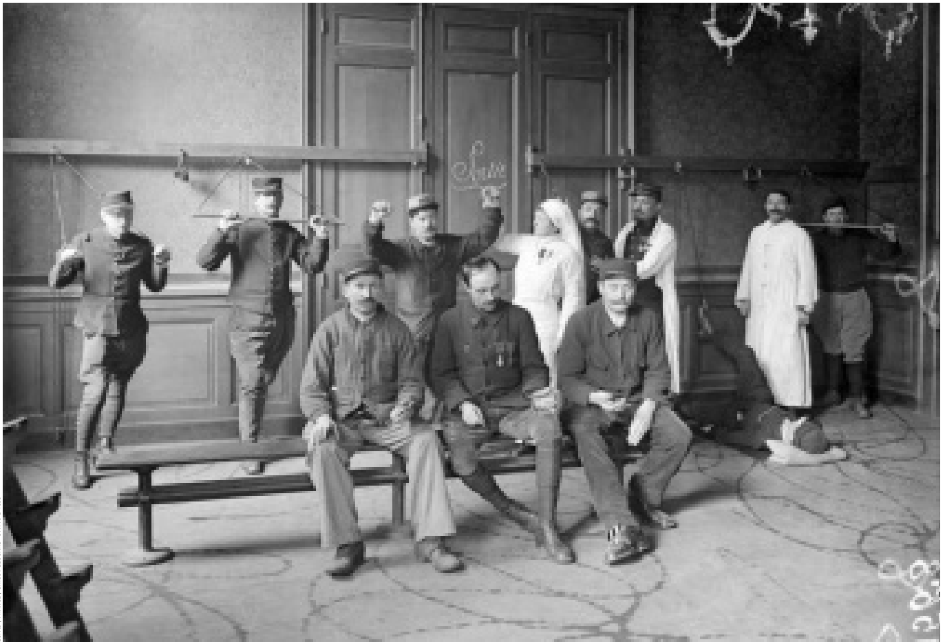
ECPAD / FRANCE / BRISSEY-EDOUARD - SPA 15 0 1988
